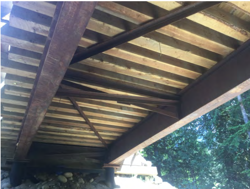
Jump span superstructure
