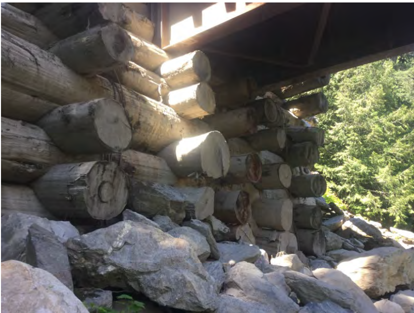
Right Bank Abutment when facing downstream
