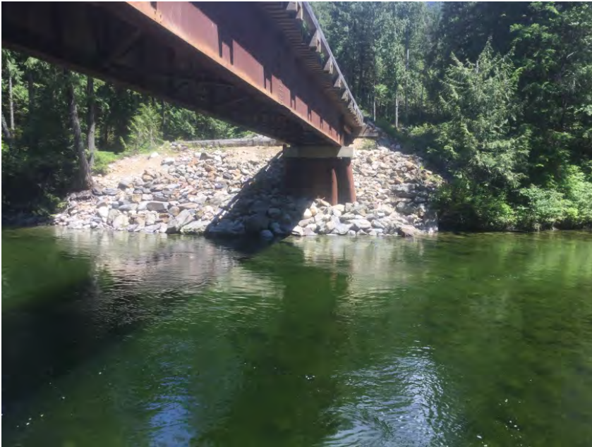
Left Bank Abutment when facing downstream
