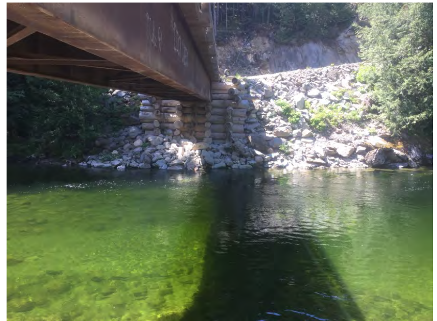
Right Bank Abutment when facing downstream
